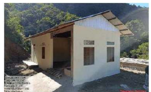
Interlocking Block Making Enterprises, Tamenglong, Manipur
